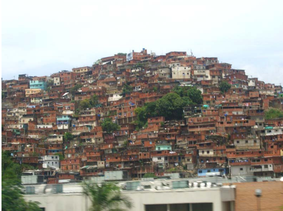
Above: The barrio of Petare, a crime-infested neighborhood on the east side of Caracas where shoddy, unlicensed building of homes continues. Petare will be featured in several scenes in Frieden's upcoming book Where Spies Go To Die .
